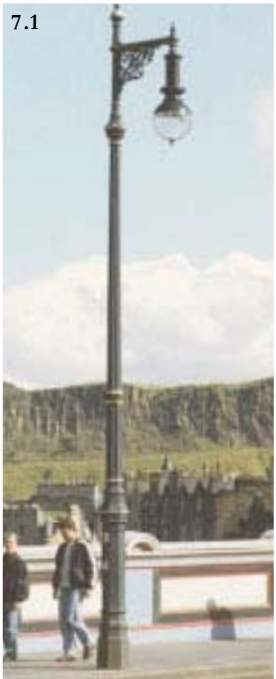
7.1 Arc Lamp 500 on Mackenzie Post, North Bridge, Edinburgh.
